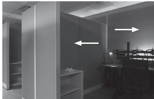
Acoustical wall treatment and partitioning
