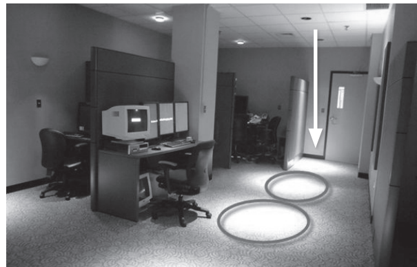
Traffic pathway lighting
